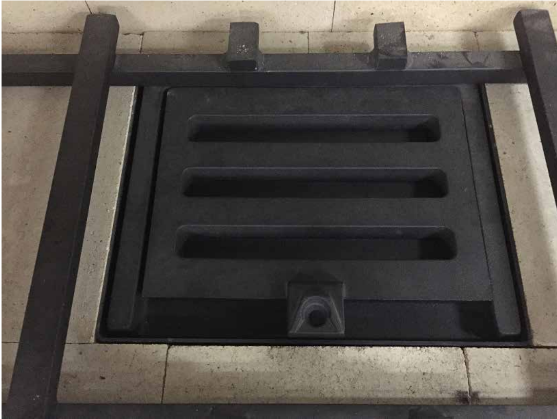
Figure 3. Both Ash Grates pictured here in the fully-closed position.
