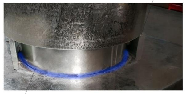
Use heat resistant sealant to seal 8" flue pipe to casing
