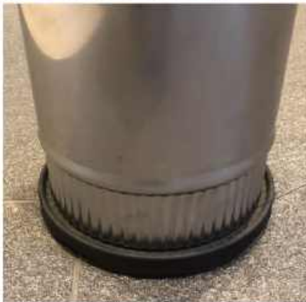
Flue seated correctly.
