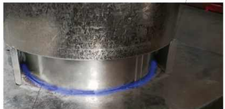
Second step in bracket stands off 10" flue pipe
