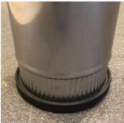
Flue seated correctly.
