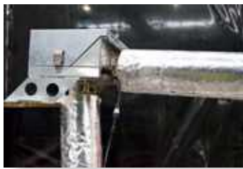
Insulation may be fitted prior and after the inline powerflue fan.
